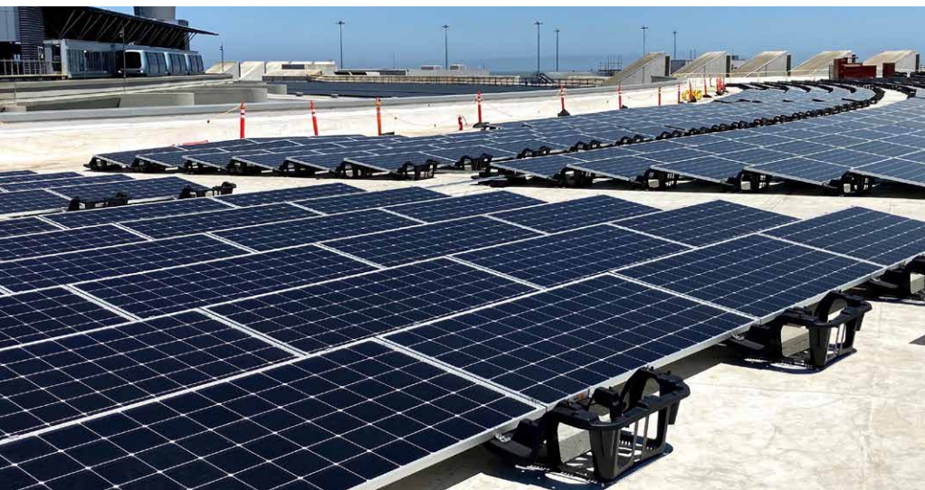
FastRack FR510-6° (above); San Francisco International Airport, Harvey Milk (Terminal 1) 1.3MW roof racking installation (left).
